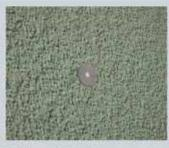
PU plugs – By insulating and sealing the anchorage point, the façade's thermal bridge is interrupted.
